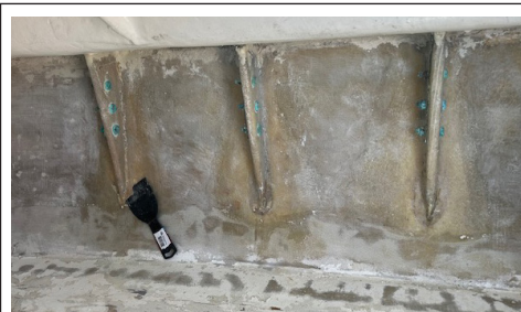
Inside View, Before
