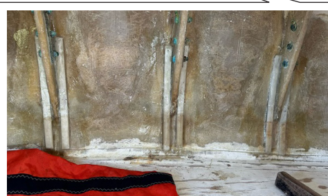
Inside View, After
