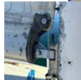
A "U" shaped bracket was added to connect the restored part to the mast.
