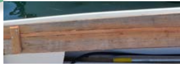
Below: A closeup of the repaired section. The center of the board had to be removed and replaced with an inlay.
